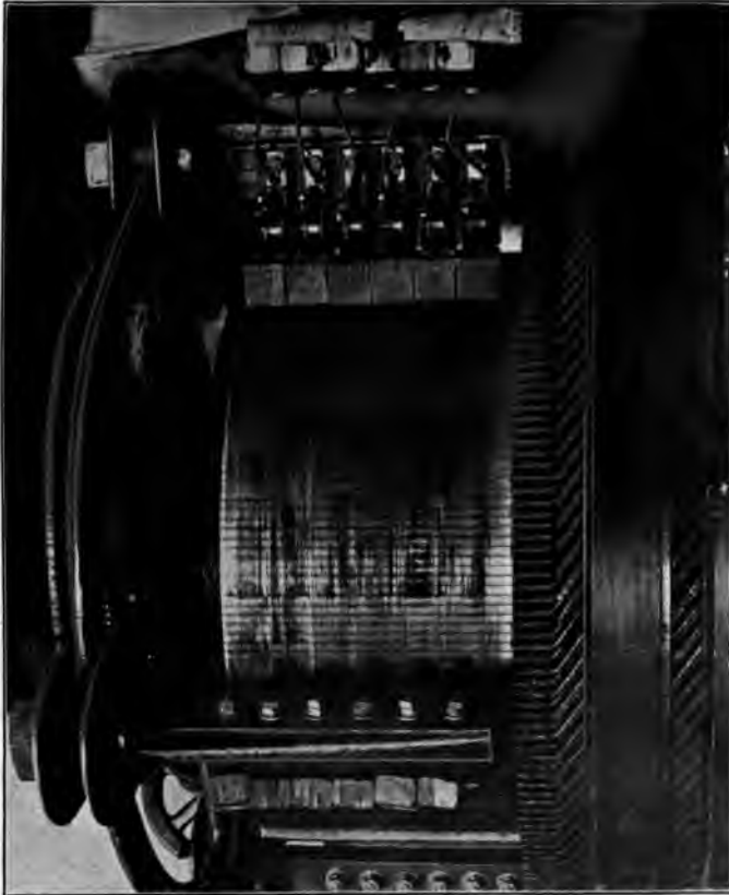
FIG. 96.—Dirty commutator surface caused by the use of a lubricant on the commutator in connection with graphite brushes. Note the collection of smut on the faces of the exposed brushes.
